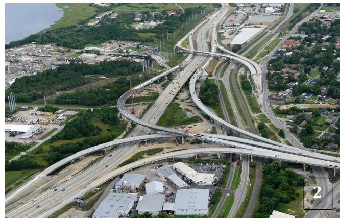
Photo 1: A current picture of Stromboli looking east from Meeting Street. When local road improvements are completed, Stromboli will connect from Meeting St., over Spruill Ave. to the new Bainbridge Connector, seen at the top of this aerial photo. Photo 2: Bridge deck construction is completed on all but the ramp from I-26 East onto the Port Access Road.
